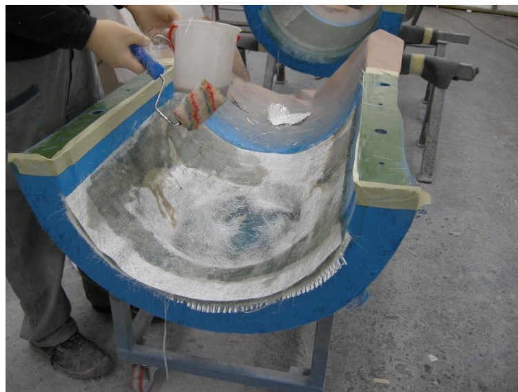
Figure 2b: A photo of the hand lay-up process at the beginning of CFR production (source: internal photographic documentation TECHNOL)
