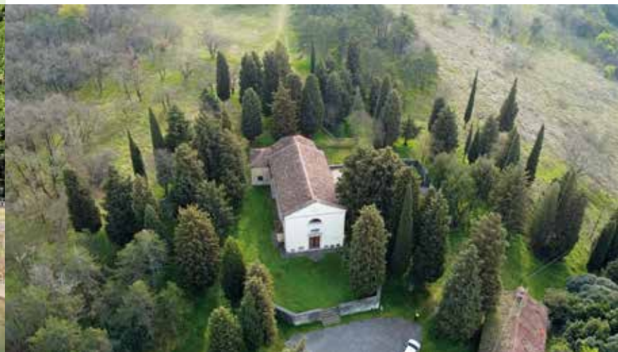
The Church of Santa Maria in Monte
