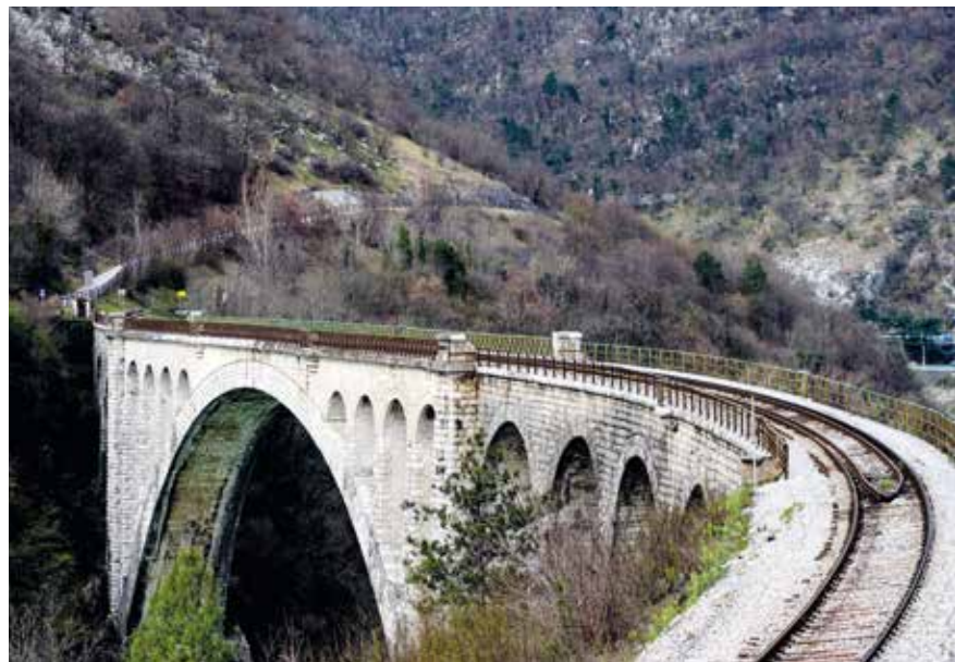
The Solkan Stone Bridge
