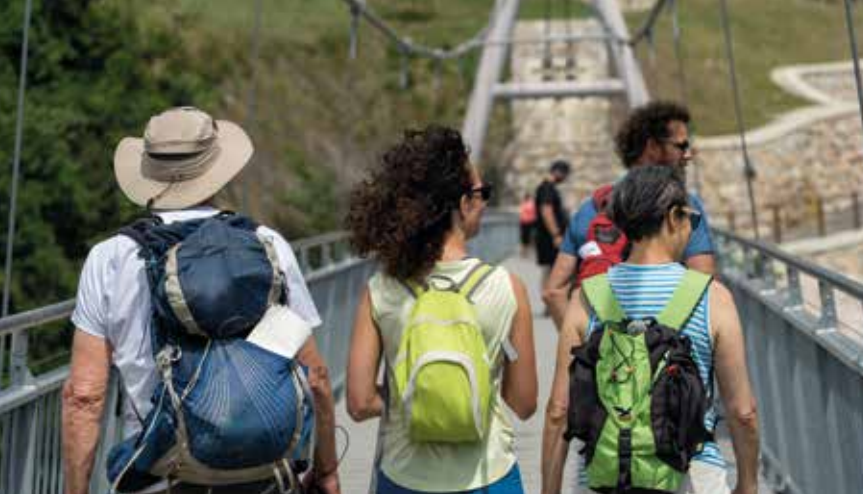
Steel pedestrian and cycling bridge over the Soča in Solkan
